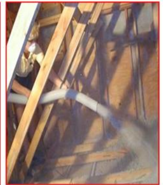
T-A-P™ insulation blown into an attic
